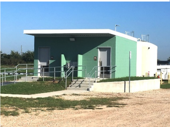
New Restroom Facility
